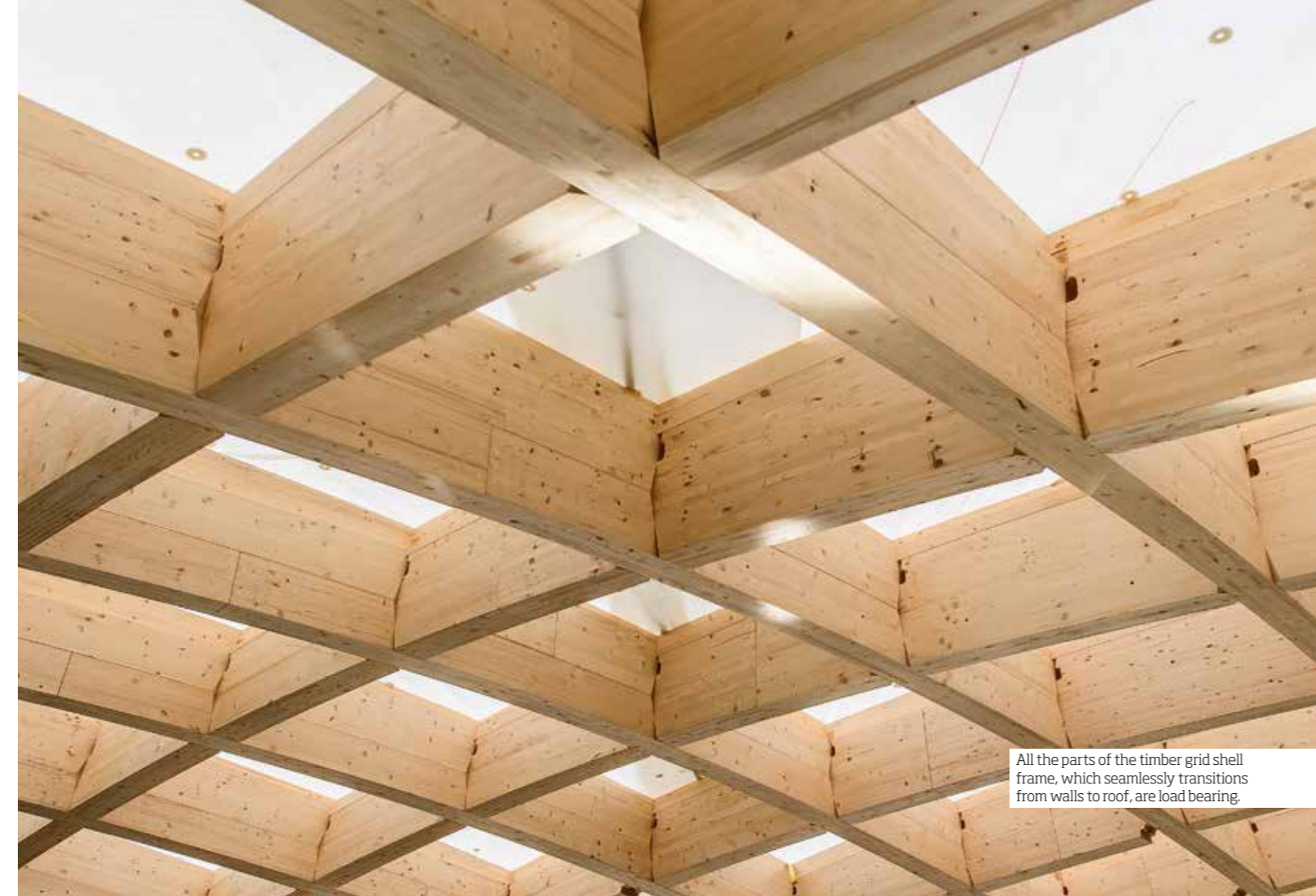
Each individual piece of wood is unique, and its exact shape only appears in one spot in the building.
