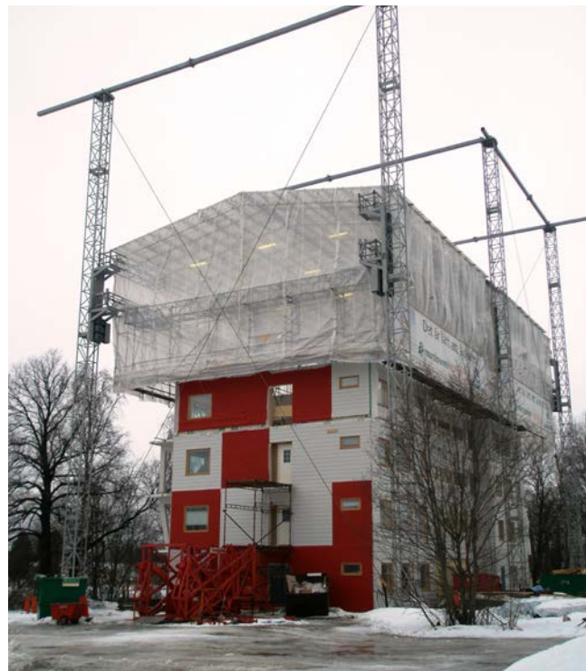
Example of climbing weather protection for dry construction with a high degree of prefabrication.
