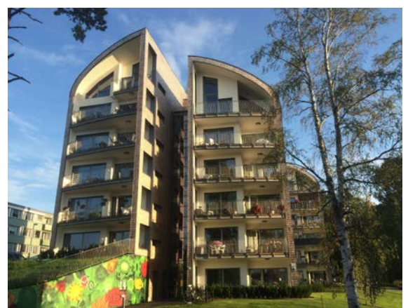
6-storey apartment block, Fristad, Sweden.
