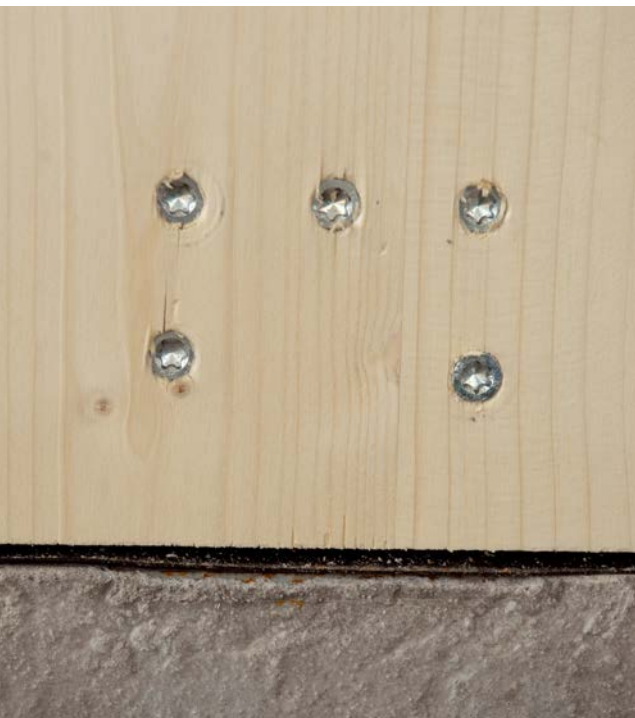
Screw joint, CLT.
