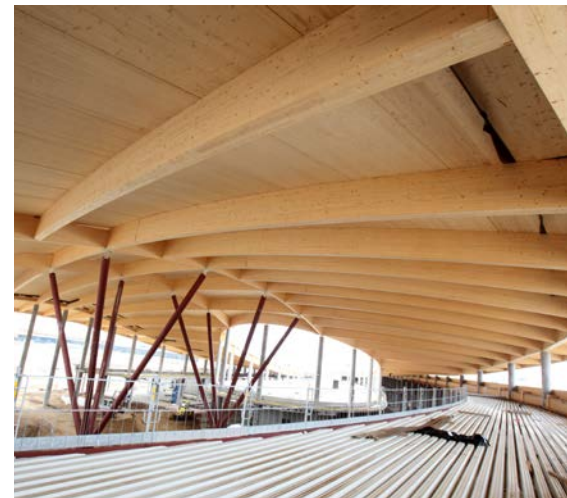
Roof made of glulam and CLT.
