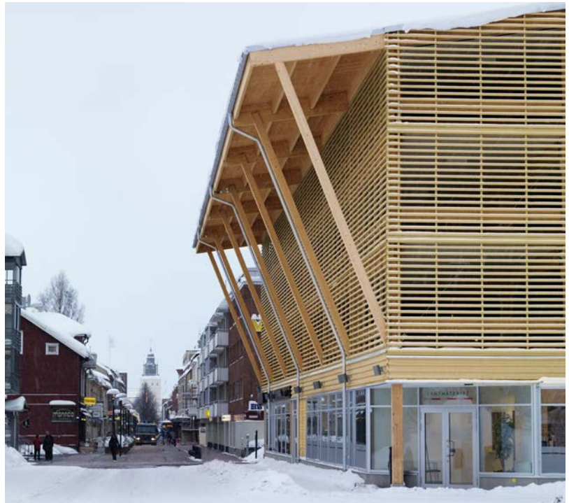
Car park with load-bearing CLT slabs, Skellefteå, Sweden.
