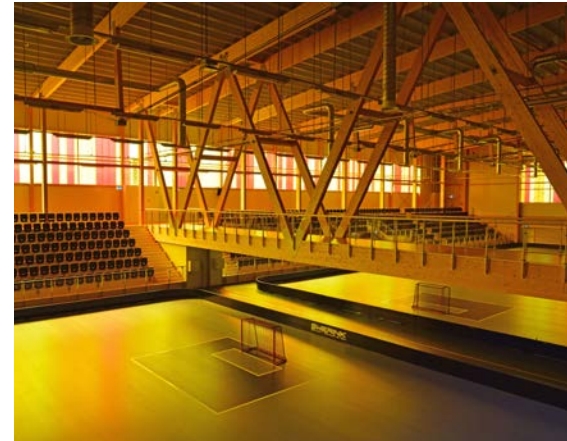
Walkway of glulam and CLT, Uppsala, Sweden.
