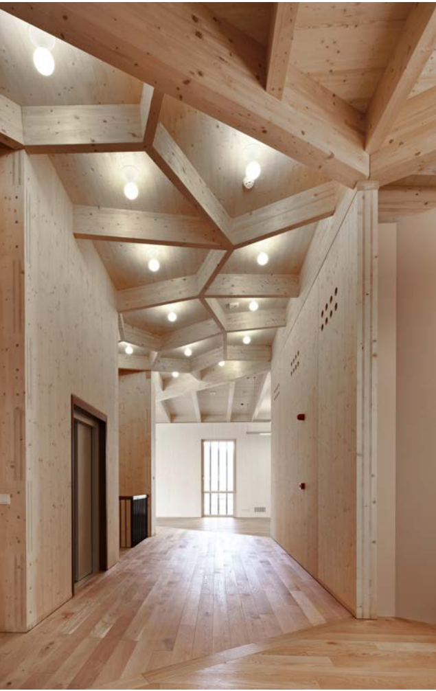
Interior with CLT and glulam beams.
