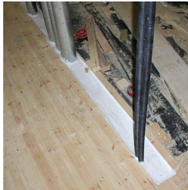
Example of sealed conduits running through a CLT floor structure.
