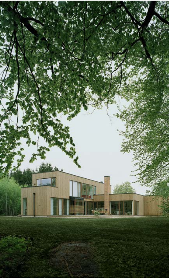
One family house made of CLT, Skara, Sweden.
