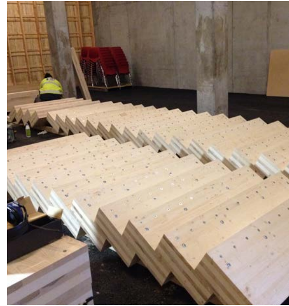
Staircases made of CLT.
