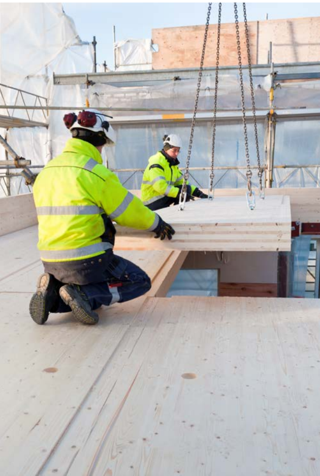
Assembly of CLT floor.
