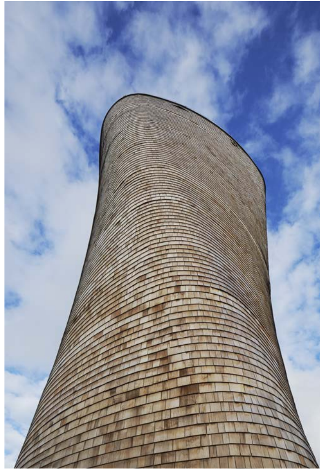
Ventilation tower with CLT frame, Stockholm, Sweden.
