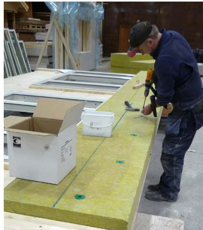
Insulation of CLT wall.
