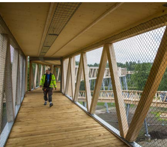
Bridge made of glulam-trusses and roof made of CLT.
