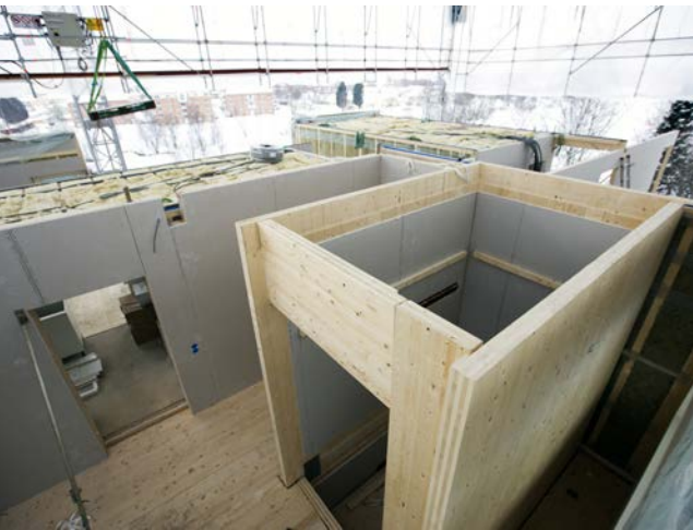
Elevator shaft of CLT.
