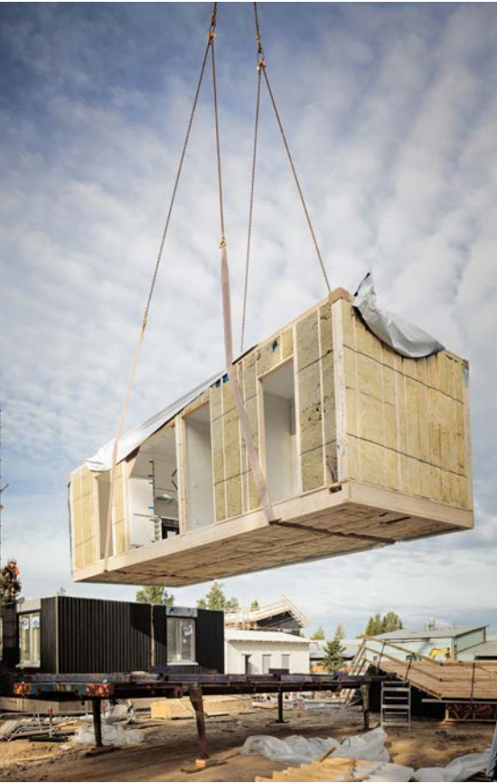
Installation of prefabricated box unit.
