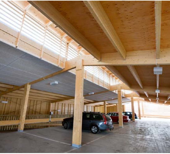
Parking structure made of glulam and CLT, Skellefteå, Sweden.
