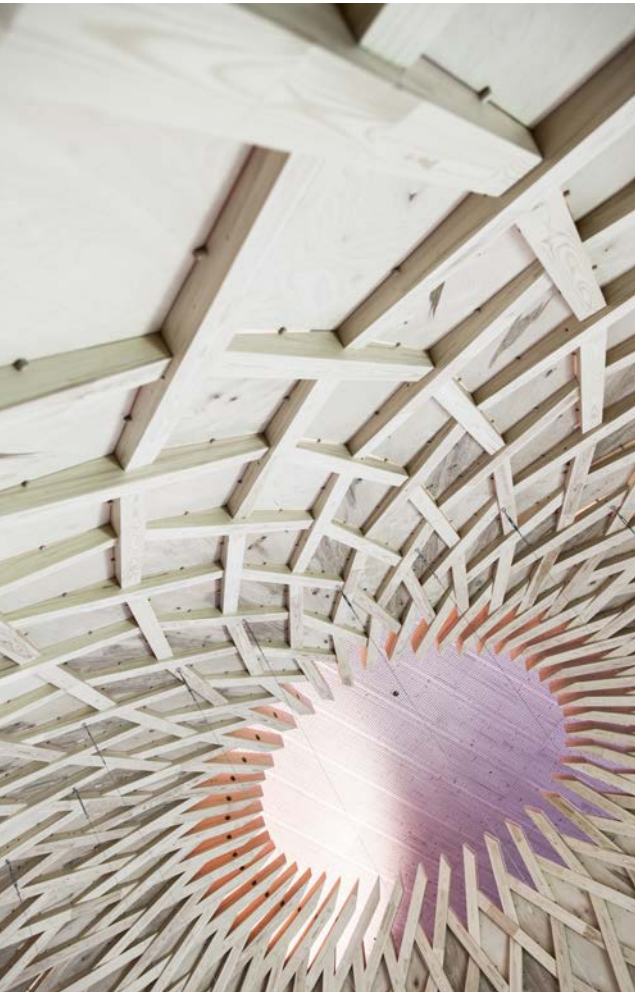
Roof made of glulam and CLT.
