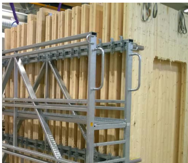
CLT panels ready for supplementary layers.
