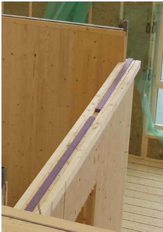
Example of a vibration-damping intermediate layer.
