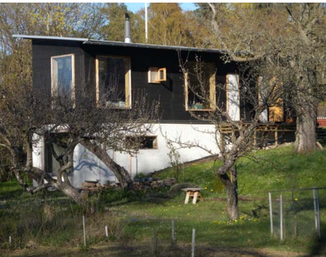
Summer house made of CLT, Öland, Sweden.
