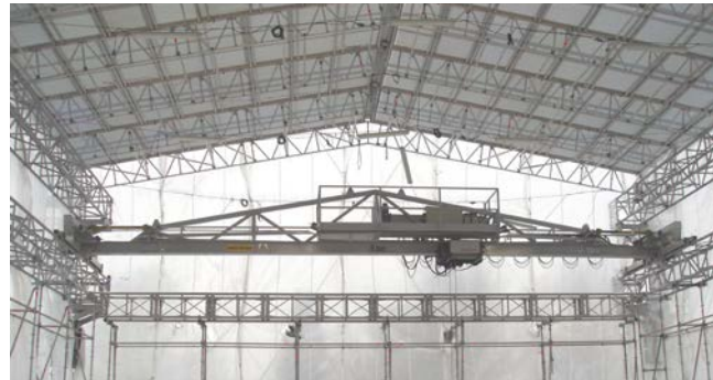
Tent with crane.
