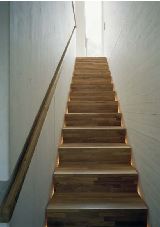
Stair with handrail milled in the CLT wall panel.
