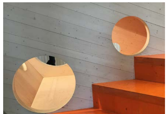
Example of holes cut in CLT. The structure of the panels provides wide scope for architectural design flourishes and adaptation to the client's wishes and requirements.
